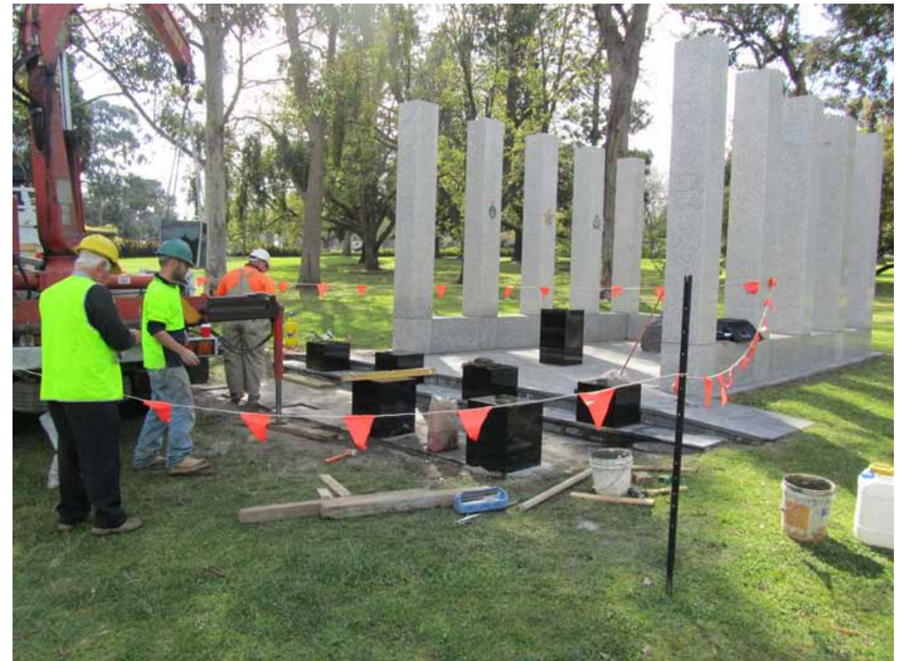
The A.H.M during the construction process.
